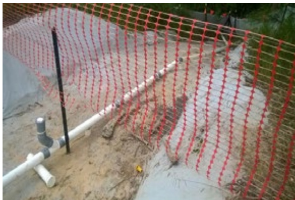
The award winning Basin Siphon Dewatering initiative
