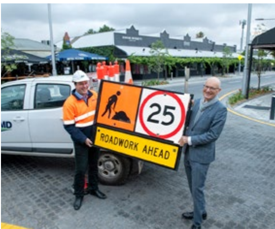
Tim Bishop, BMD Construction Manager and David Pisoni MP, Member for Unley remove the project's last construction sign
