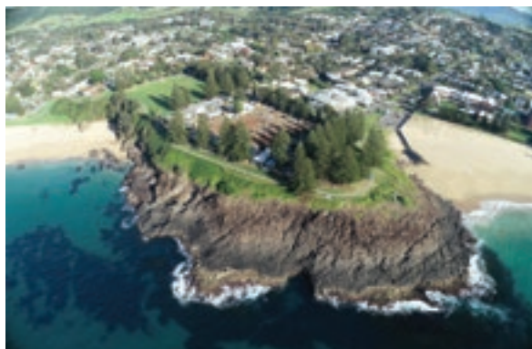
A still drone image taken at the Kiama Surf Beach Holiday Park project in New South Wales
