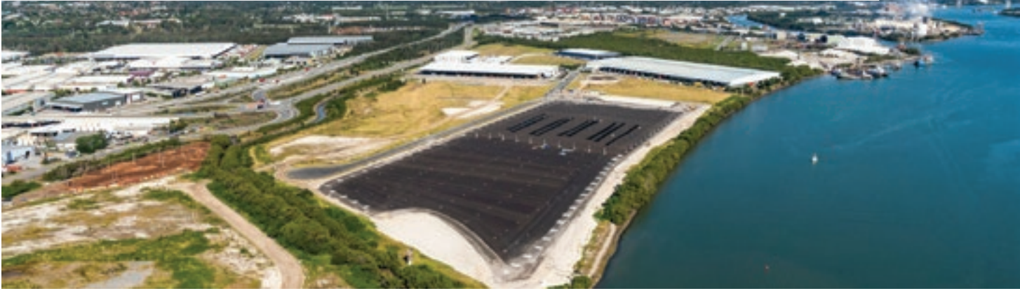
Autocare Car Storage Area project, Port of Brisbane
